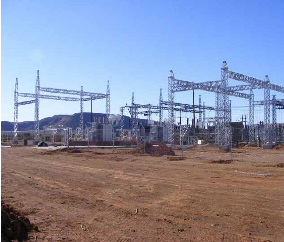
Above: Upgrade of Karoo substation from 5MVA to 10MVA capacity
