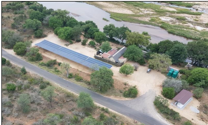
Nkuhlu solar PV plant (Photo: SANParks)
